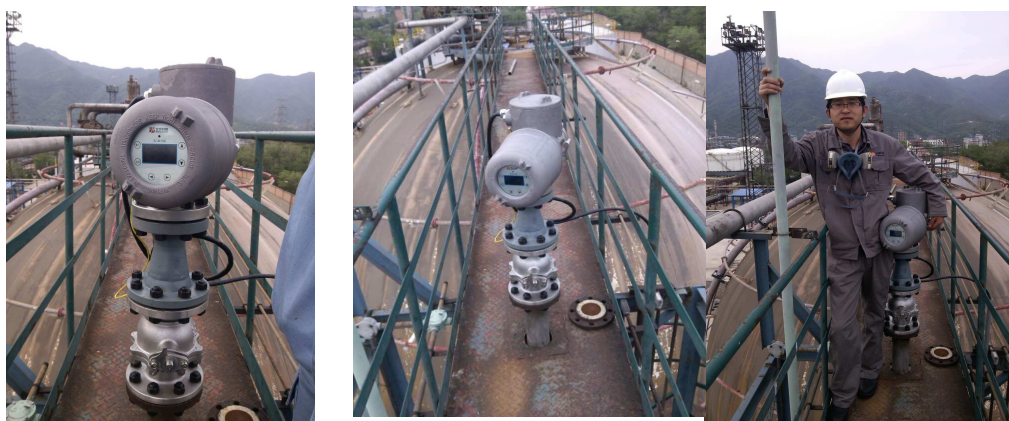
Diagram of servo tank gauge installed outside Spherical pressure tank
